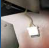
Untidy holes where after-make items have been removed
